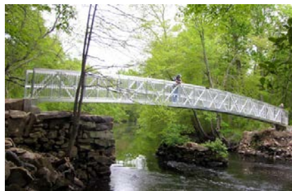
The new Polly Coon Bridge over the Pawcatuck River
